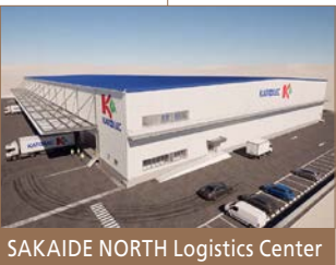
SAKAIDE NORTH Logistics Center
